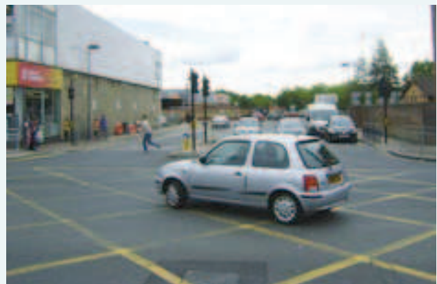
Junction on Station Road with the shopping centre access road
